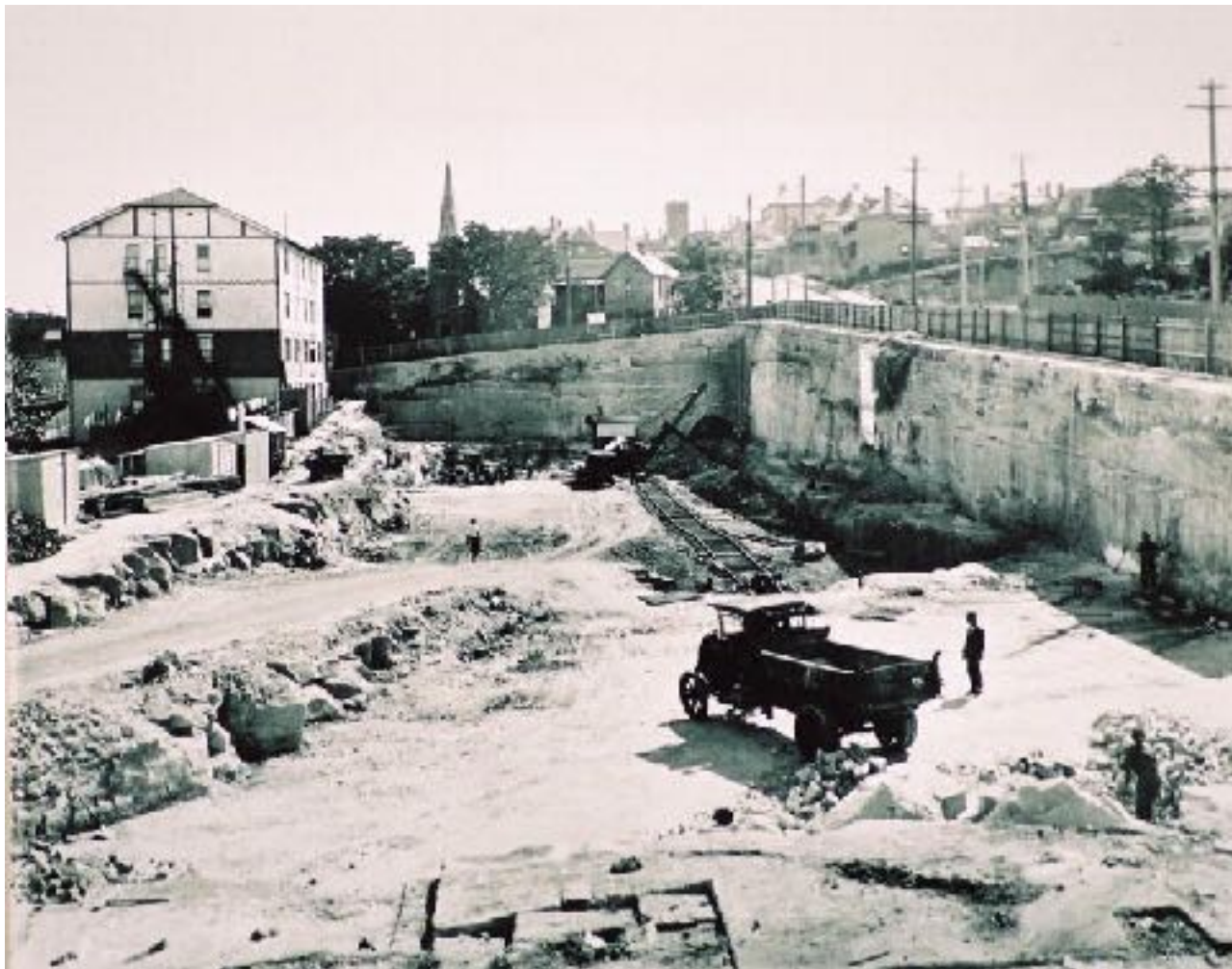
Construction of Railway Tunnels and Station at North Sydney 1920 - Heritage centre North Sydney Library (Note Holtmann's Tower and St Peter's Church Spire in the background)
