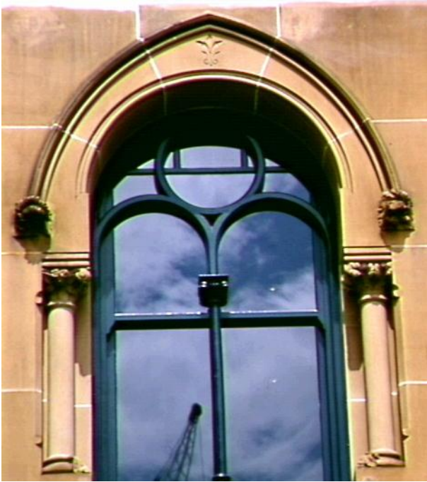
Figure 72 – Sandstone elements on facade, 1991-92. Source: City of Sydney Archives, NSCA CRS 904/1209
